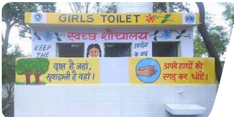
New Toilet Construction Work has been completed in GPS Bhigan
