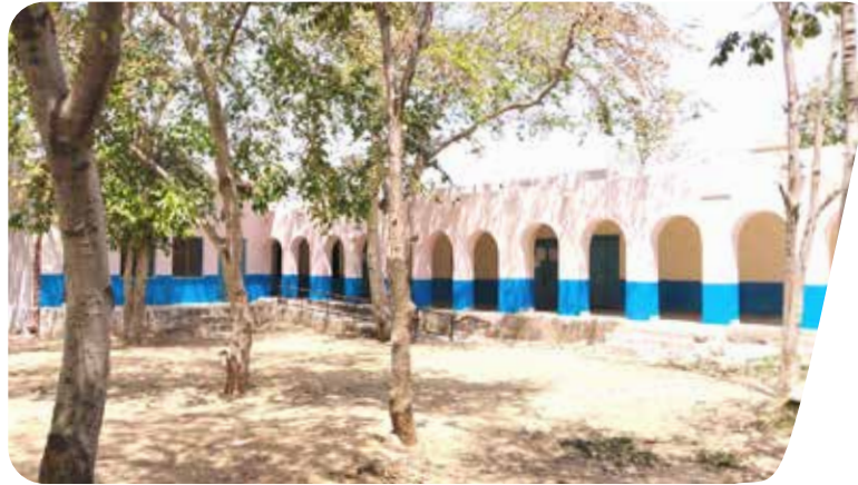
Whitewash is completed in Neemrana School
