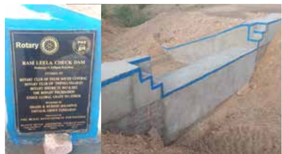
Construction work on check dams has been completed
